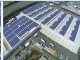
Saitama Plant, Glass Bottle Company (Saitama Prefecture)
