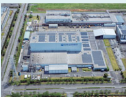
Utsunomiya Plant, Plastics Company (Tochigi Prefecture)
